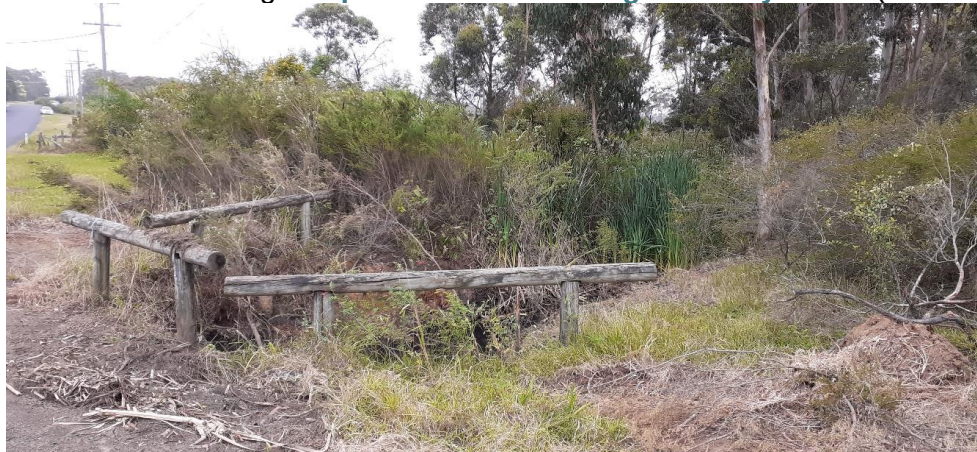
Figure 17 Existing Southern Culvert/headwall at Sealark Road-North up
